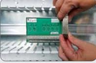
Then routes the cable through the wire duct and snaps the other end of cable to the 1492 IFM Module.
